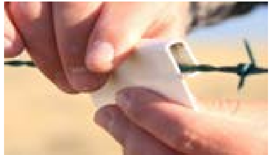
Installation of visual fence markers.
