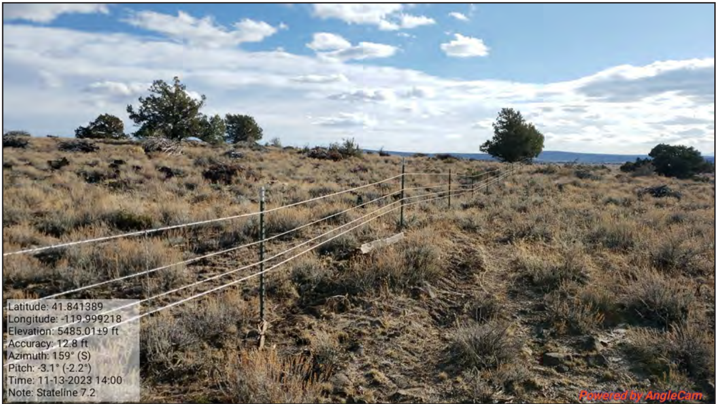
Figure 15. Stateline Fence during final project inspection.
