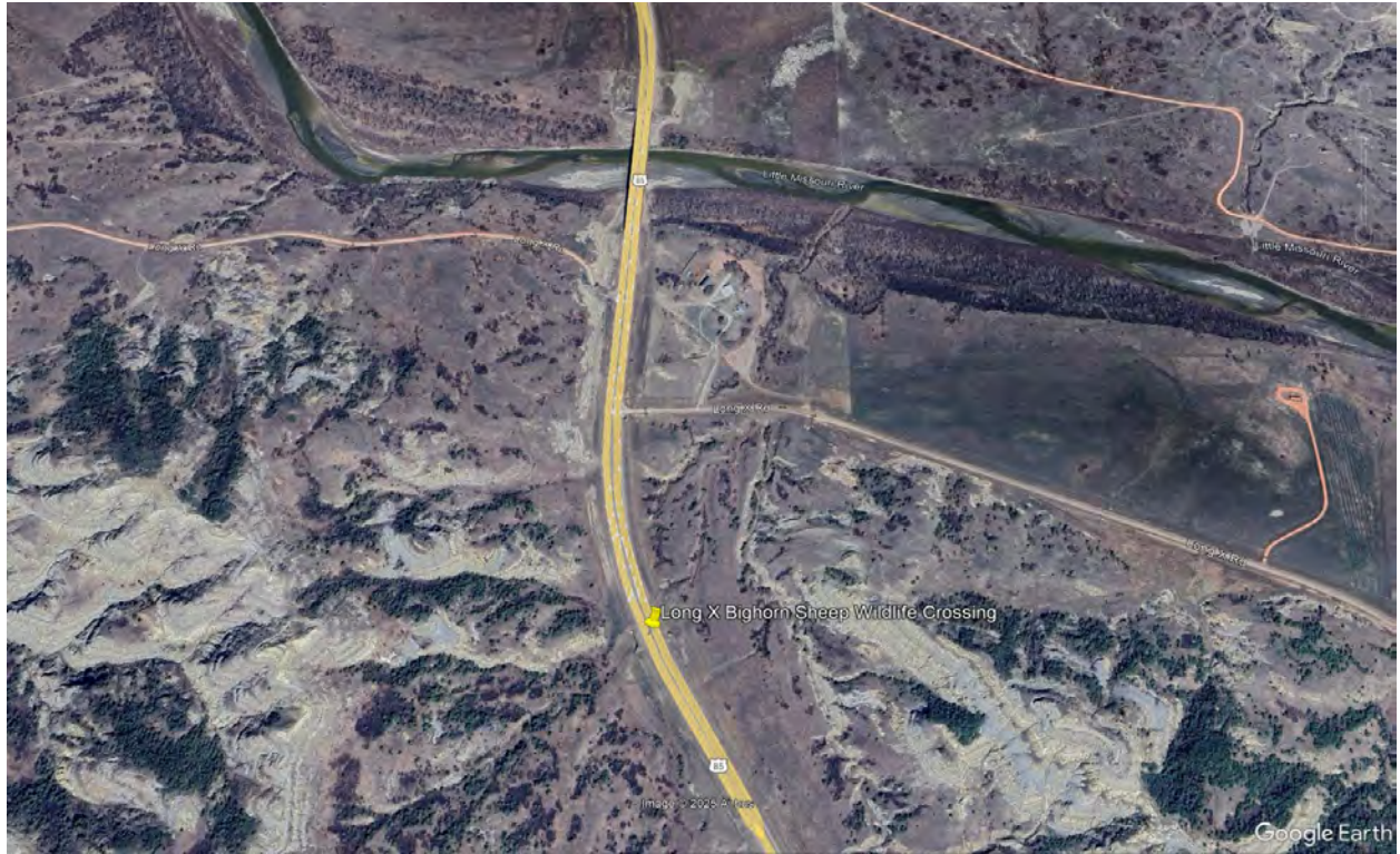
Figure 6. Aerial image of the Long X bighorn sheep wildlife crossing location south of Watford City, ND.
