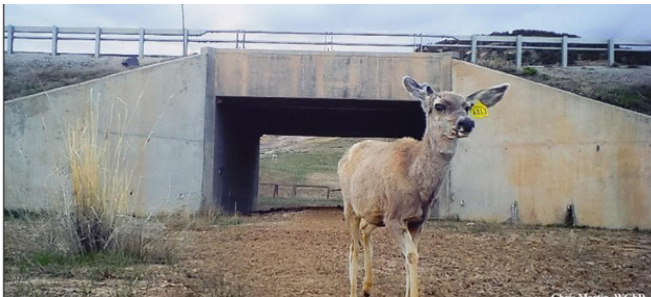
A mule deer doe successfully uses an underpass to navigate under Wyoming Highway 789.
