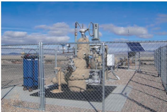
*After drilling, a fenced well casing and control equipment is left in place like this structure at the Salt Wells Geothermal well site near Fallon, Nevada (operated by ENEL North America, Inc.). Photo courtesy of Bureau of Land Management, Nevada State Office.*
