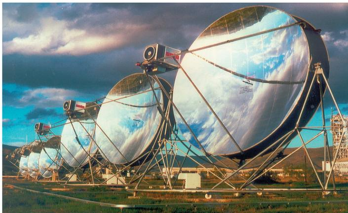
*Each of these Dish/Engine units produces 10 kW of power. (Photo courtesy of Sandia National Laboratory)*
