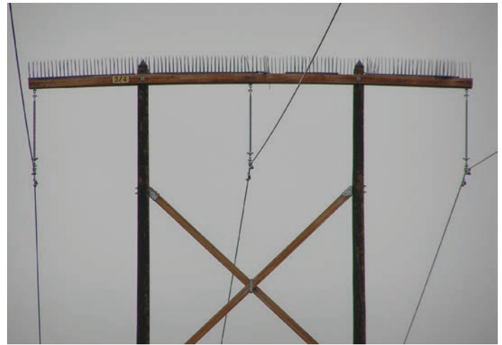
Figure 18. Managers should be aware perch-deterrent devices discourage, but do not always eliminate perching by raptors and corvids, especially in areas where natural perches are limited. Perch-deterrent devices need only be installed on problem structures, such as those located immediately adjacent to a lek or within key nesting and brood-rearing habitats. (Photo by M. A. Schroeder/WDFW).
