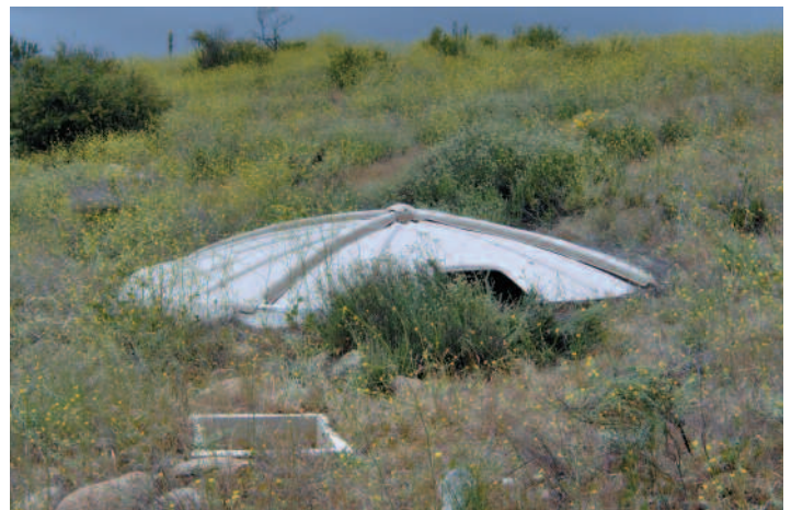
Figure 29. Upland game guzzler modified to provide water for deer. Note trough in lower left corner is connected to the guzzler to maintain water level (Photo by Randy Botta/CDFG).
