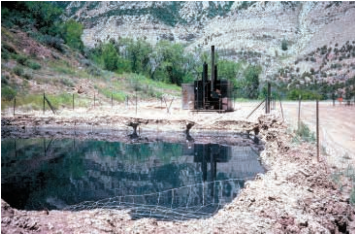
Figure 53. Improperly fenced collection pits pose risks to wildlife in search of water. (Photo courtesy of CDOW).
