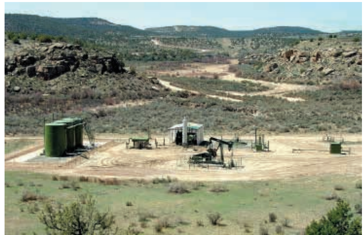
Figure 48. A typical gas well; 1-2 acre footprint. (Photo courtesy of NMDGF).
