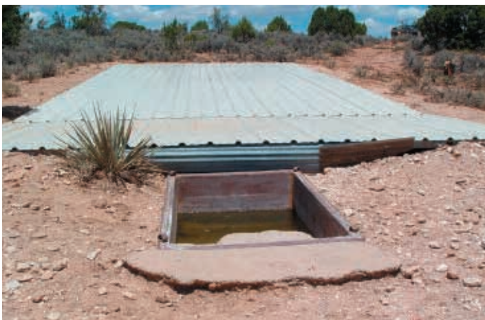
Figure 40. Big game water catchment and drinking tank in Northern Arizona. (Photo by Luke Thompson/AGFD).
