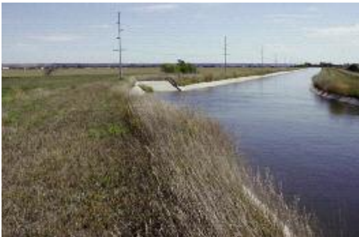
Figure 17. Diversion canal built with concrete ramp to provide escape for trapped animals. (Photo by Bruce Trindle/NGPC).
