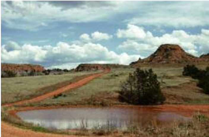
Figure 16. Professional assistance is frequently needed to design water structure systems to match storage capacity to estimated watershed yield. (Photo Mike Blair/KDWP).
