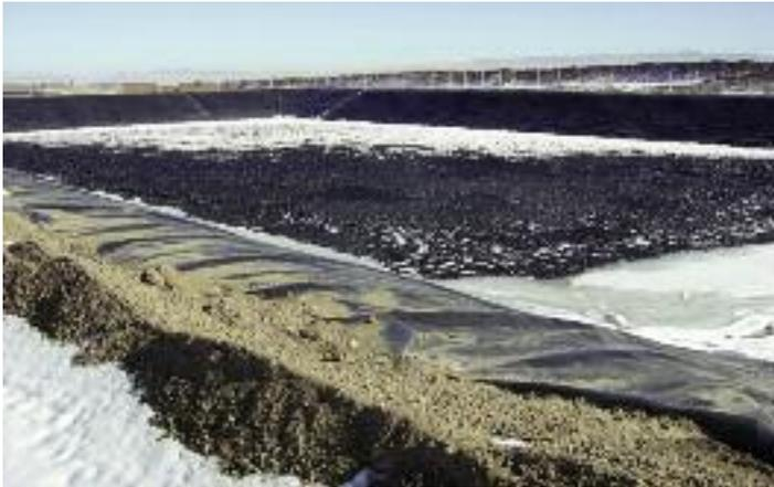
Figure 62. Process pond with deer exclusionary fencing and bird balls, Humboldt County, NV. (Photo courtesy of NDOW).
