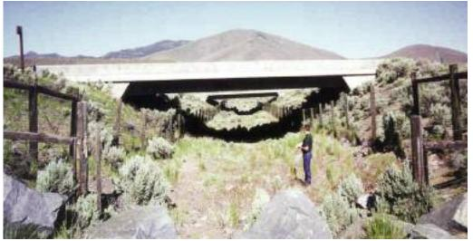
Figure 68. Highway underpass wildlife crossing on 4-lane stretch of U.S. Highway 395 in northeastern California, fenced to direct migrating deer safely under the roadway. (Photo by Mike Cox/NDOW).
