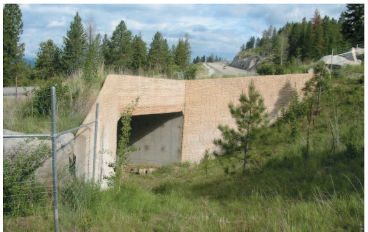
Figure 37. Locate wildlife passage structures to take advantage of terrain features. Steep terrain restricts the entrance way of this passage structure. Also note the use of fencing and boulders to guide deer movements. (Photo courtesy Wayne Wakkinen, IDFG)
