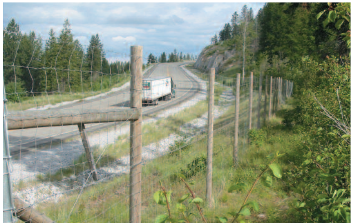
Figure 36. Ungulate-proof fencing can reduce collisions, improving human safety and mule deer survival. Care, however, must be taken to avoid blocking migration routes, or fragmenting habitat for mule deer or other wildlife species. (Photo courtesy of Wayne Wakkinen, IDFG)
