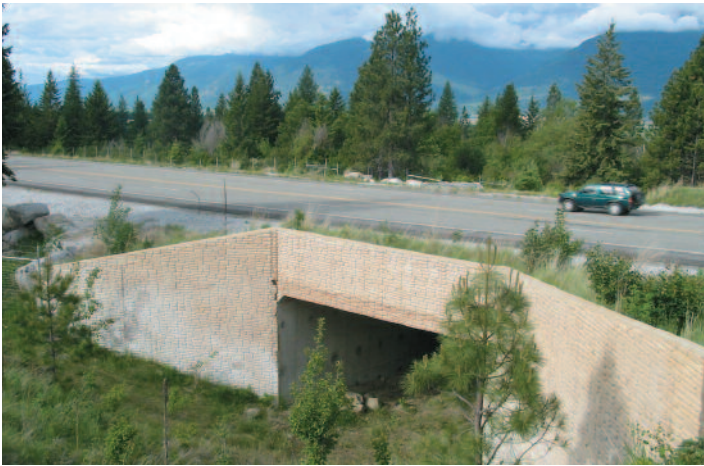
Figure 34. Wildlife underpasses provide permeability for travel corridors, allowing seasonal use of an area, and movement through the area during migrations. To encourage use, locate structures near existing deer travel corridors and away from human activity. (Photo courtesy Wayne Wakkinen, IDFG)
