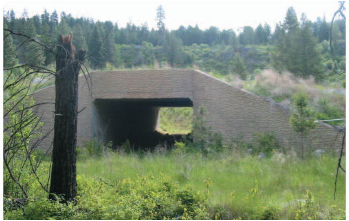
Figure 35. Level terrain near the entrance of this wildlife structure encourages use by wildlife and allows wildlife to see through the structure from either end. (Photo courtesy Wayne Wakkinen, IDFG)
