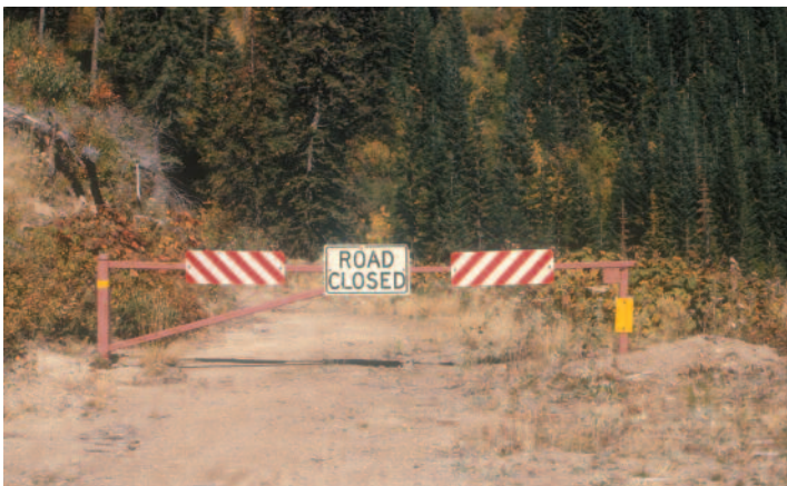
Figure 15. The post-logging strategy for road management should be part of the initial sale design, with temporary roads signed as such. Gates, barriers, and road re-contouring should be used where appropriate to maintain less than 1.9 miles of open road per square mile. (Photo courtesy IDFG)
