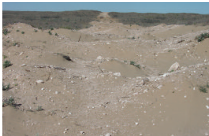
Figure 45. Maintenance roads to service oil wells should be reclaimed by disrupting the soil and making the road impassible in conjunction with reclamation protocols that ensure habitat recovery to the extent possible (Photo courtesy of NMDGF)
