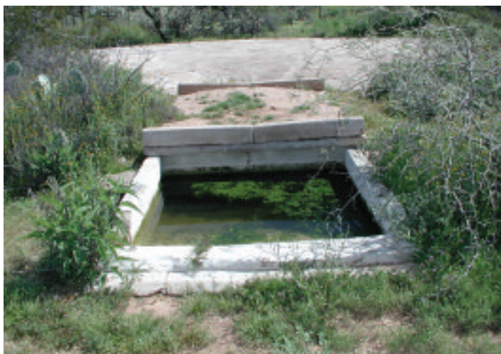
Figure 26. A water catchment with collection apron and drinker can be built anywhere in mule deer habitat using any one of a multitude of designs. Catchments should be designed to have as little visual impact on the environment as possible (Photo courtesy of Mike Demlong/AGFD)
