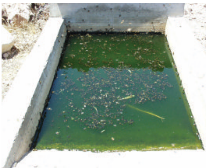
Figure 25. Although water quality in artificial catchments rarely affects the health of the animals using it, these water sources should be maintained as free from organic debris as possible. (Photo by S. Rosenstock/AGFD)
